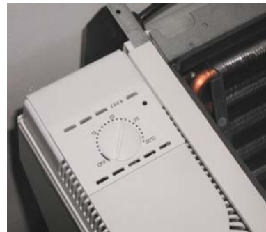
ANALOGUE CONSOLE INSTALLED ON A FAN COIL UNIT
